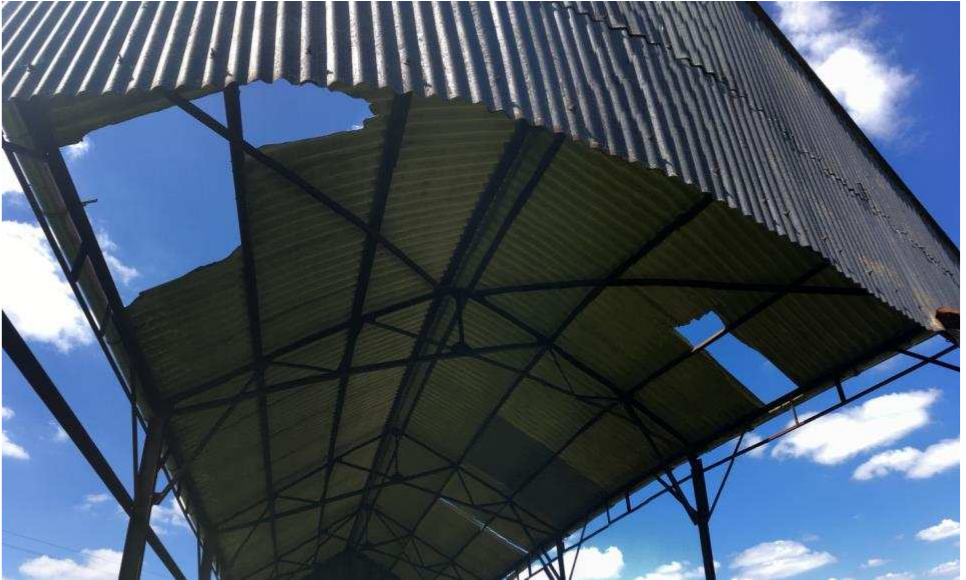
View of roof of Barn No. 2
