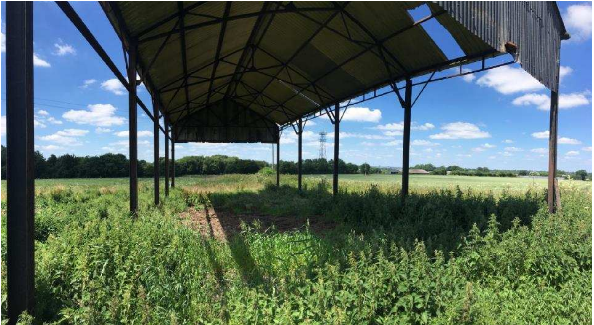
View inside Barn No. 2
